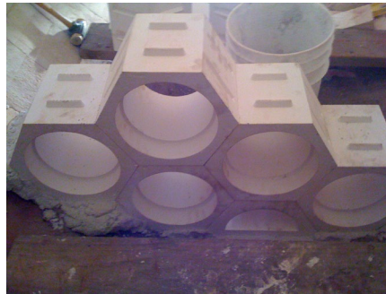
Blocks are locked together at installation
