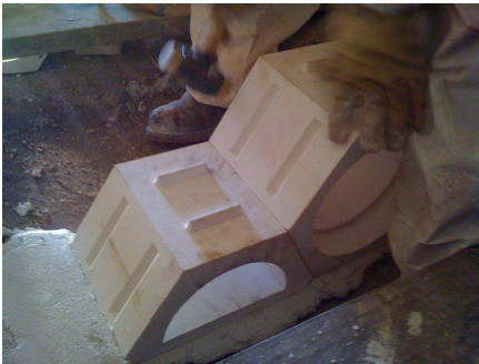
Alternating tabs and slots on each side
