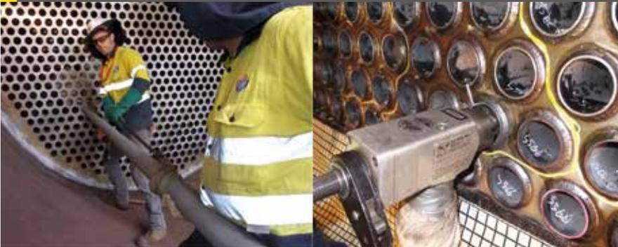
Fig 6: Marking out hand holes prior to complete removal
