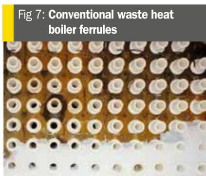
Fig 7: Conventional waste heat boiler ferrules
