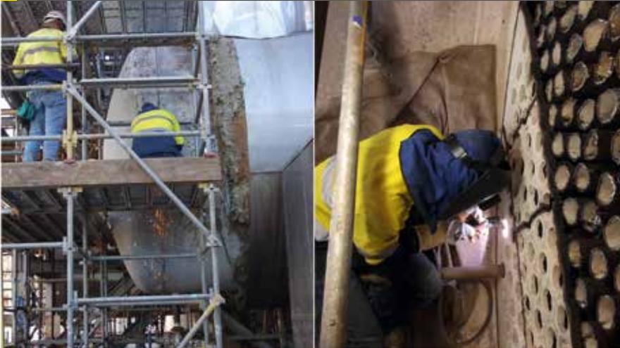
Fig 4: Hot end tube cutting
