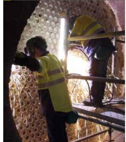
Fig 5: Insertion (left) and cutting (right) of new tubes
