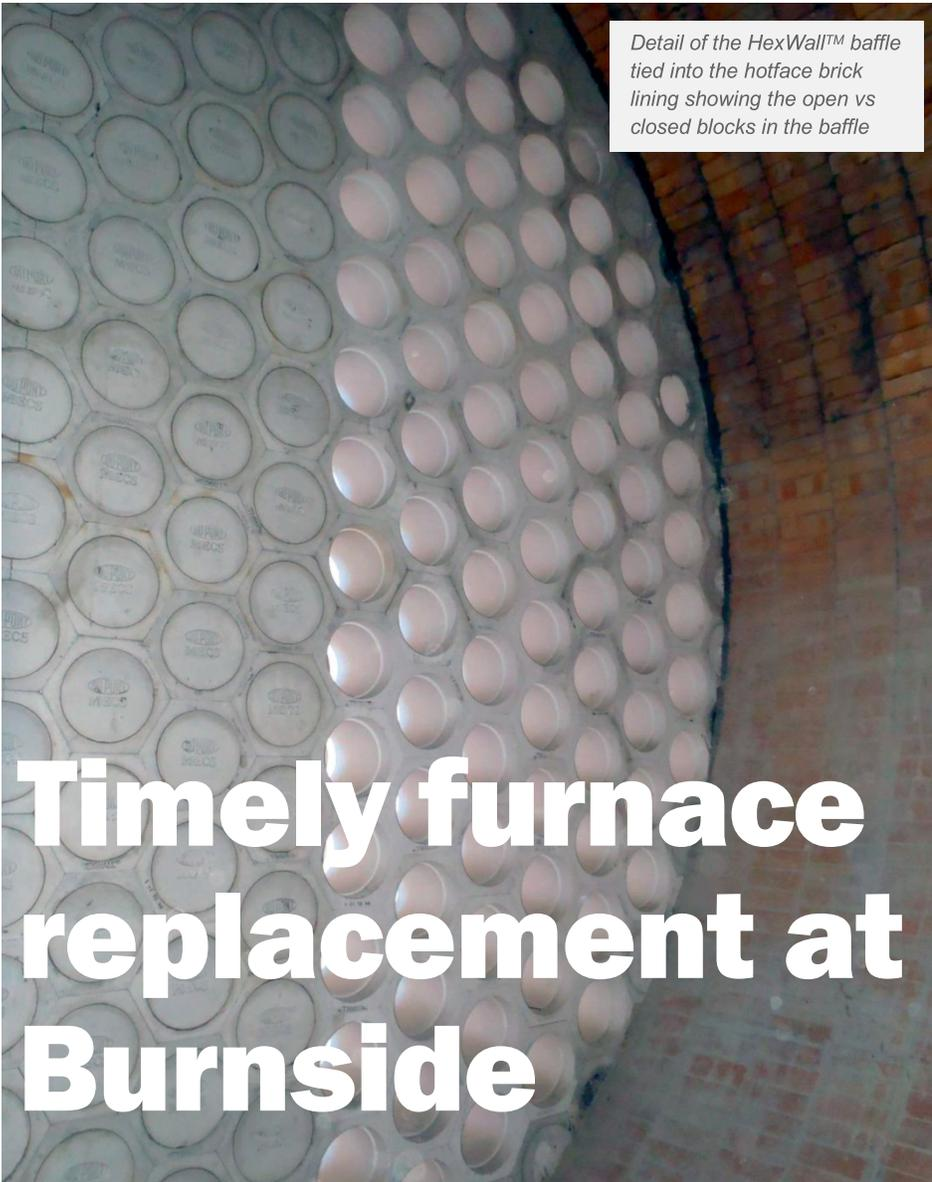
*Detail of the HexWall™ baffle tied into the hotface brick lining showing the open vs closed blocks in the baffle*
