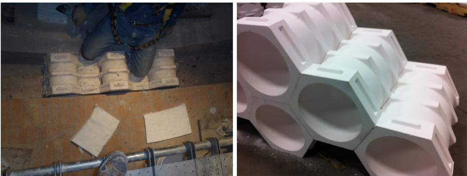
**Figure 9:** MECS® HexWall Installation
