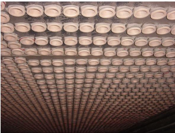
**Figure 2:** Ceramic tubular air heater inserts were installed at this coal-fired power plant to eliminate erosion of the inlet.
