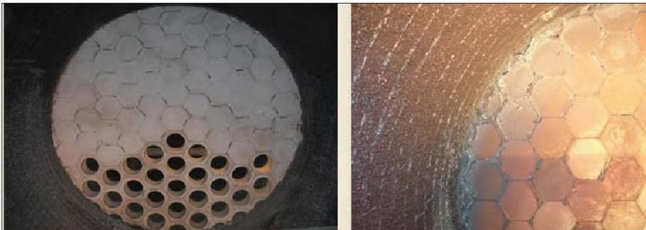
Figure 12: New HexWall (left) and after five years' service (right) in the Borderland plant
