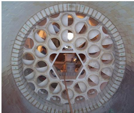
Figure 2: Newly installed hex block VectorWall
