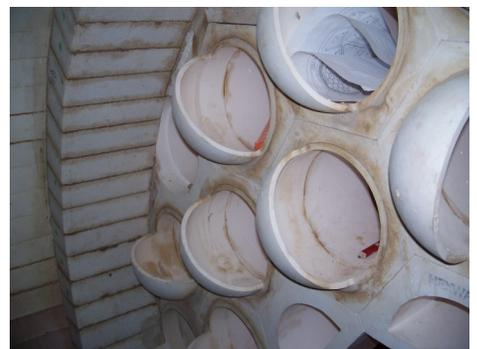
Figure 3: VectorWalls with the flow vectoring inserts clearly visible
